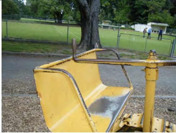
Sharp edges, Crush point Head entrapment gap
