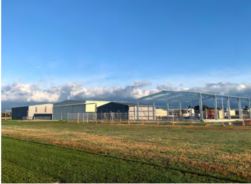
Figure 2: Tranche 1 hangar construction in April of 2021
