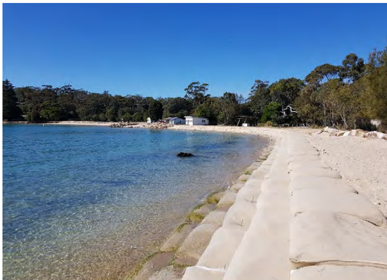
Figure 68: Example of a GSC revetment in NSW, Australia (Geofabrics, accessed 2023)
