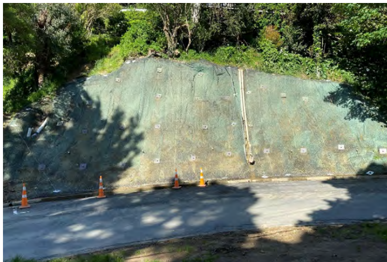
Figure 6-15: Example photograph of anchor and mesh slope remediation
