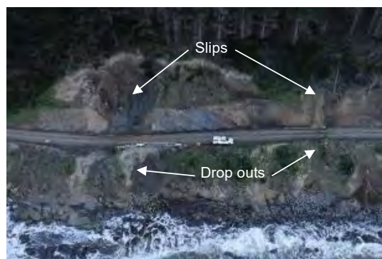
Figure 3-8: Slips and dropouts on approach to Te Rarena o Te Aohuruhuru (Suicide Rock) 27
