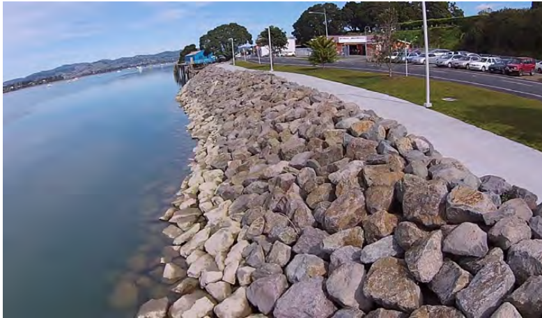
Figure 6-7: Example of a rock armoured revetment at Tauranga (Cirtex, accessed 2023)
