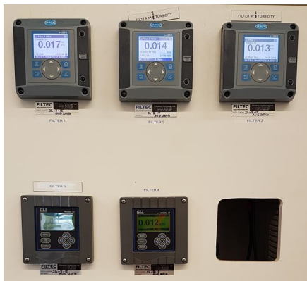
Figure 13. Turbidity readings for each filter
