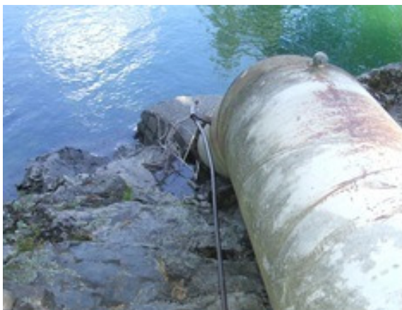
Figure 5. Waingawa River siphon intake
