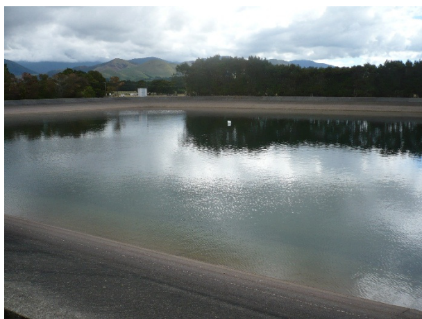
Figure 7. Raw water storage pond 1
