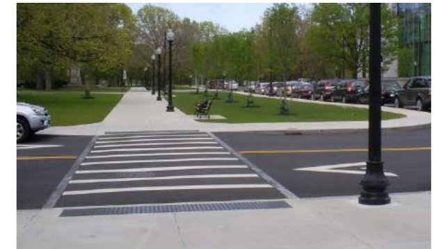
Examples of street crossings
