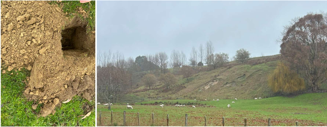
Photos 5 and 6: Soils on 6e4 (left) and the unit itself (right). Note the extensive erosion and trees for mitigation.
