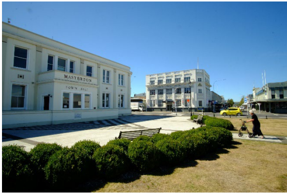
Figure 7: Wide angle view across the Plaza illustrating the relationship between the Town Hall and Municipal Buildings to the Ex-Public Trust building (note this photograph is taken from within the historic alignment of Perry Street to the front of the Town Hall).
