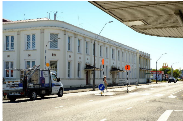
Figure 2 : Chapel Road frontage
