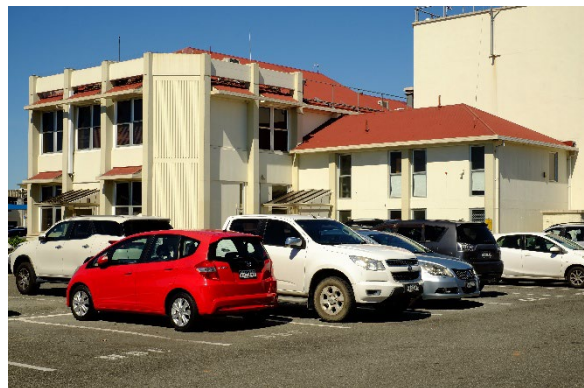
Figure 4: Northeast elevation (civil defence building)
