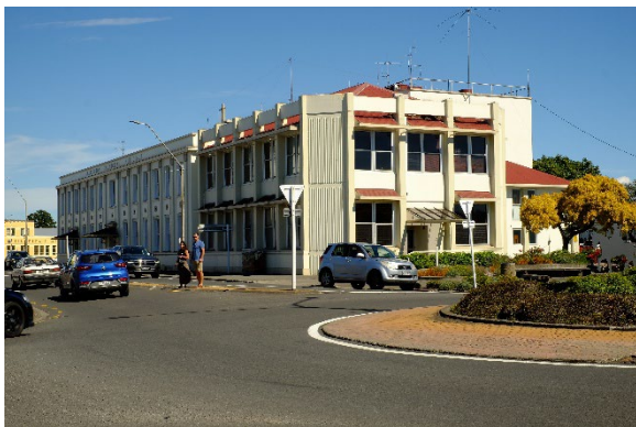
Figure 3: Northeast elevation (civil defence building)
