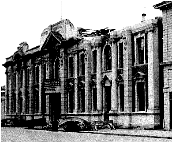
Figure 7 – Post 1942 earthquake showing minor damage.
