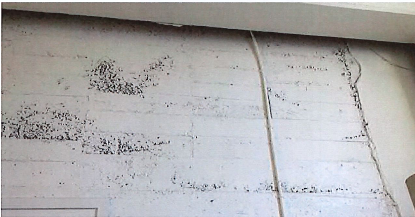
Figure 11 – View of hall extension "boney" concrete – poorly vibrated concrete resulting in exposed aggregate.
