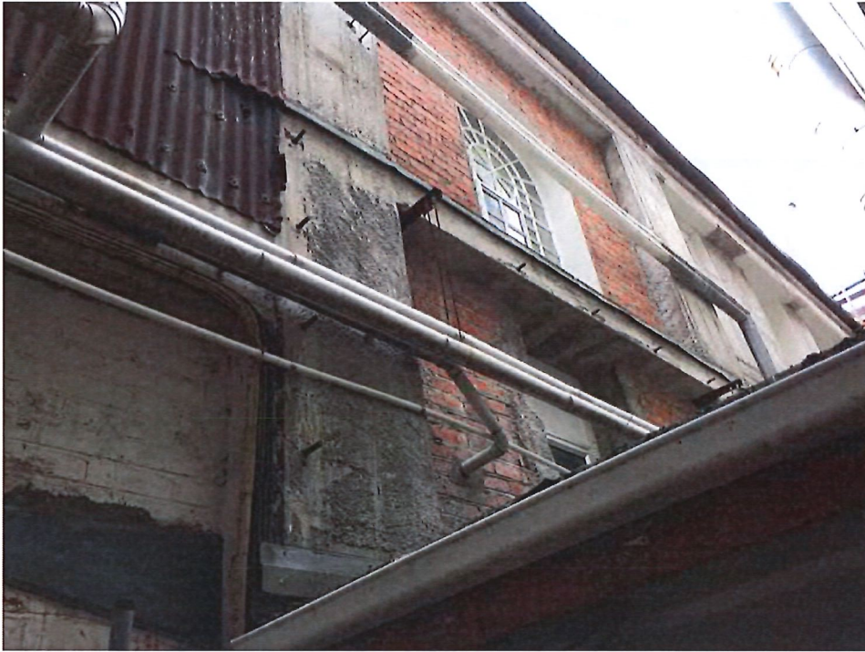
Figure 15 – External view of wall line at rear of Municipal building (shown in red in figure 13)
