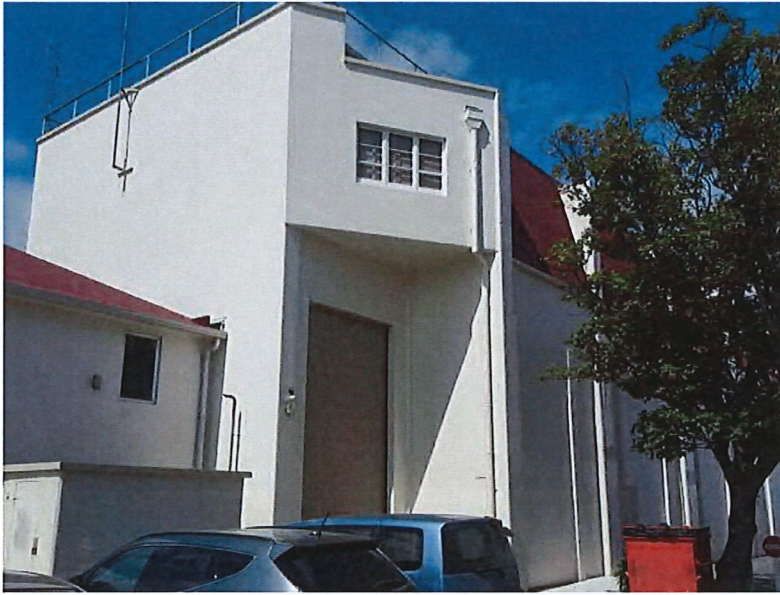
Figure 10 – Rear of Hall showing reinforced concrete extension
