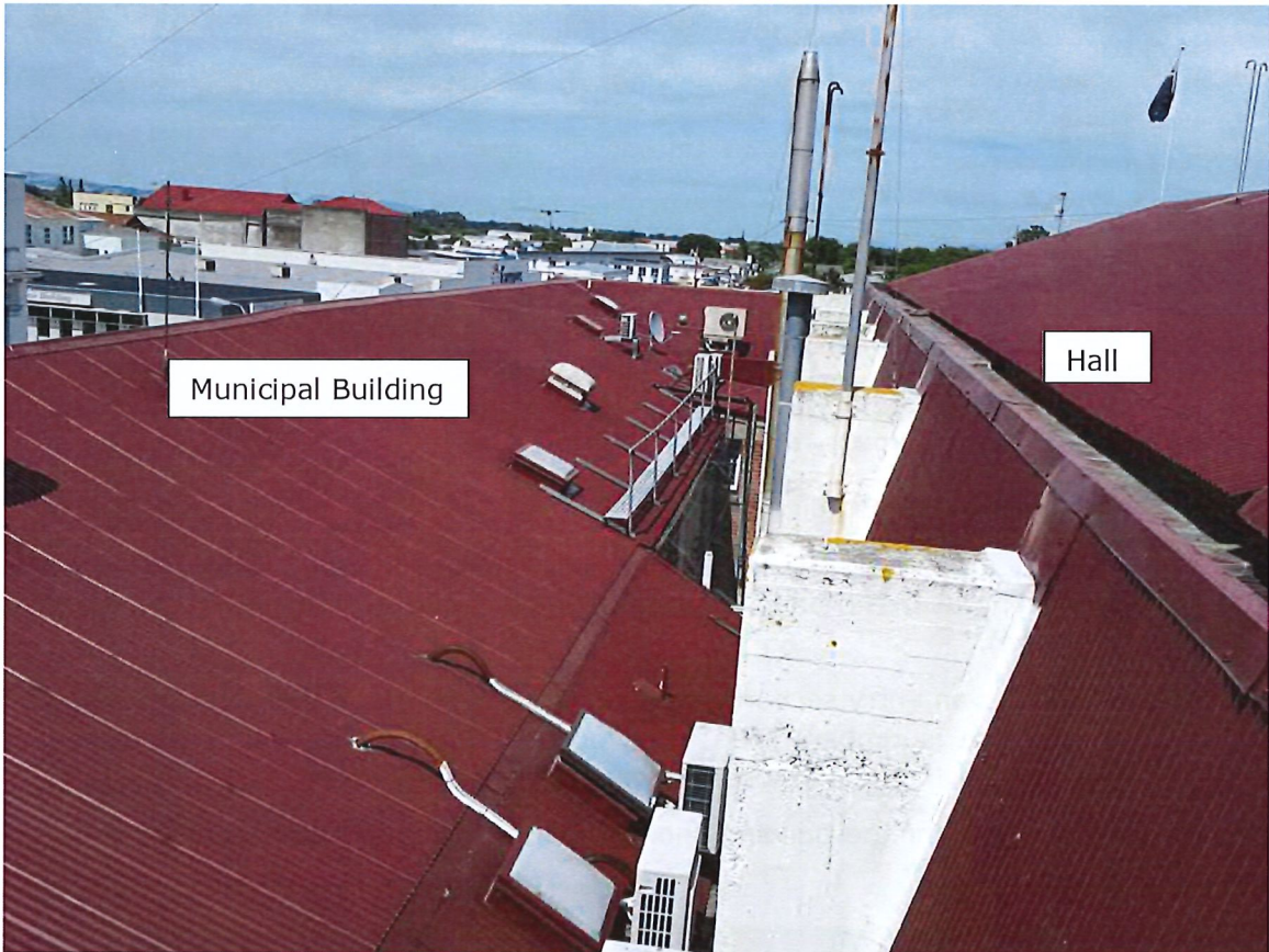
Figure 6 – Photo of roof – note space between the Hall & Municipal Building
