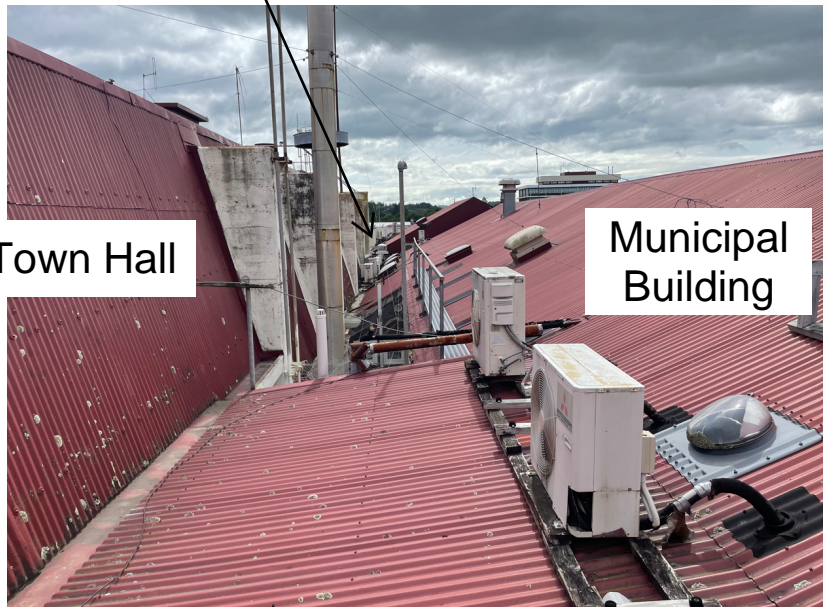
View along east wall
