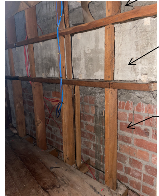
View - South wall
