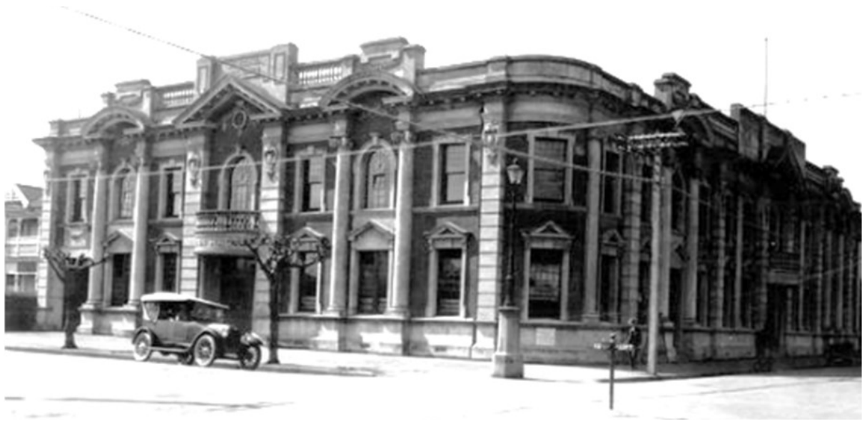
Figure 4 - Town Hall in 1930 before the 1942 earthquakes
