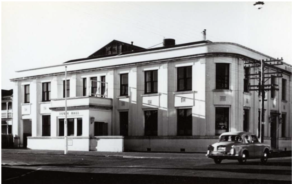
Figure 5 - Town Hall in 1954 following completion of work to repair the 1942 earthquake damage
