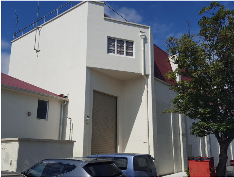
Figure 10 – Rear of Hall showing reinforced concrete extension
