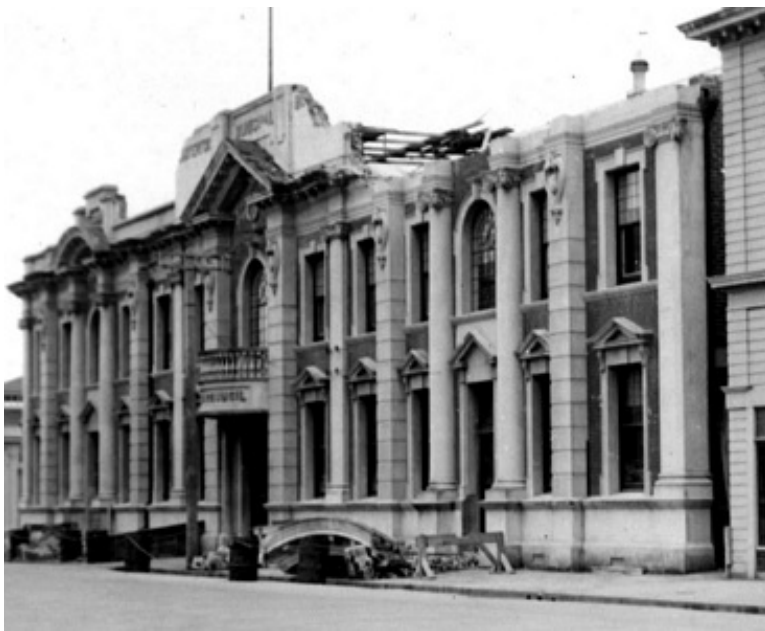
Figure 7 – Post 1942 earthquake showing minor damage.
