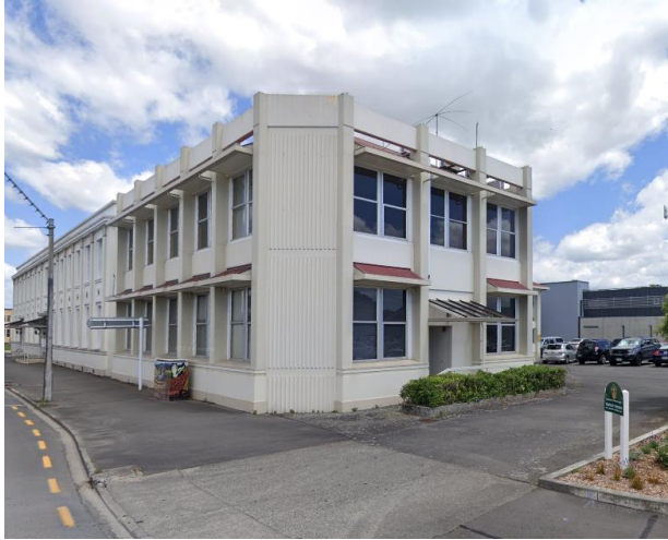
Fig 5: Existing Civil Defence Building
