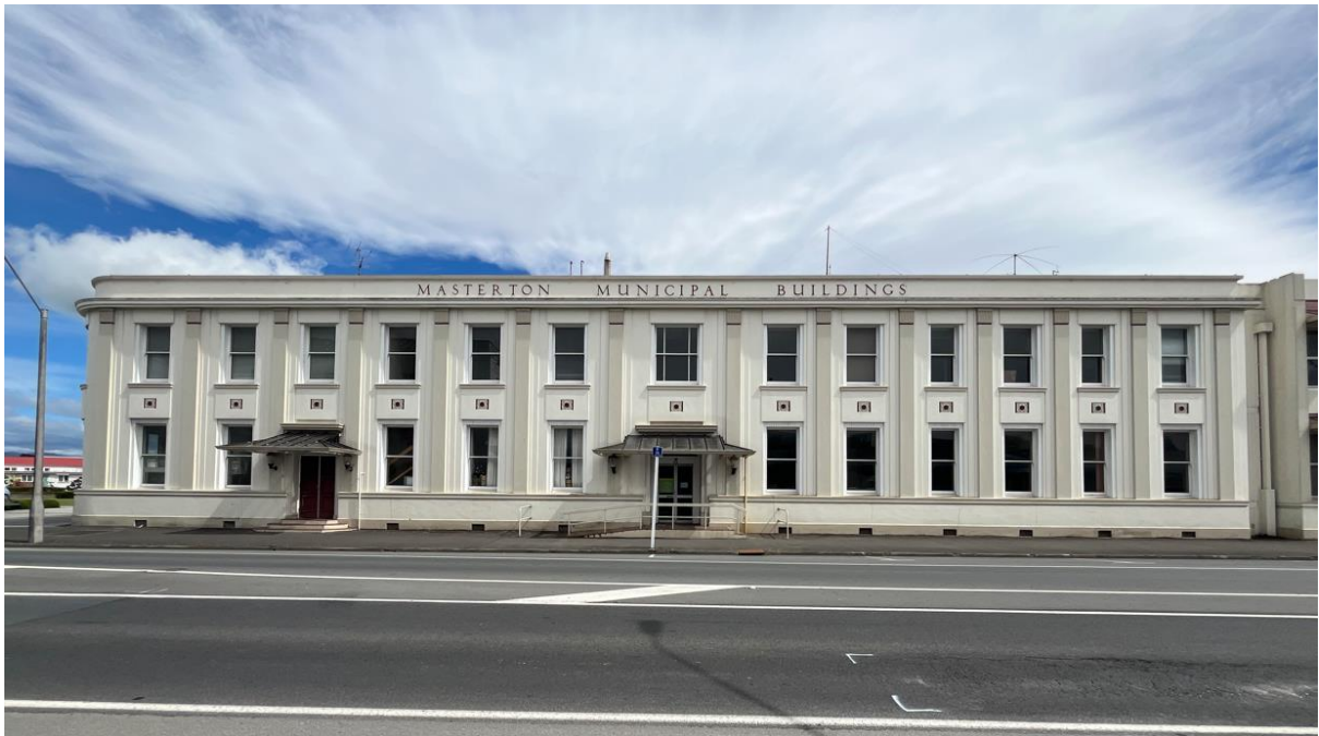
Fig 4: Municipal Building Chapel Street Side Entrances
