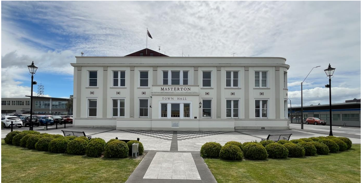
Fig 3: Municipal Building Façade with Town Hall main entrance in foreground.
