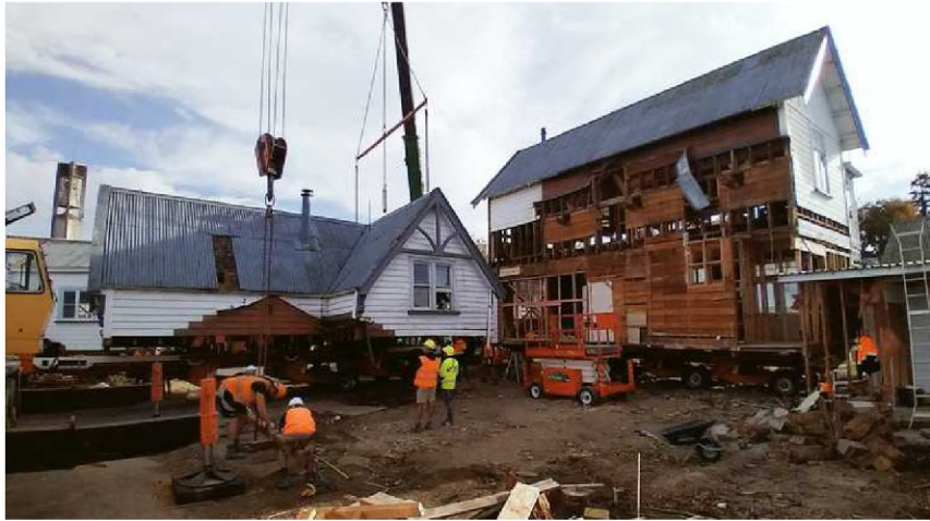
Illustration 8: Building removal in progress (4th April 2022 Chessa Stevens)
