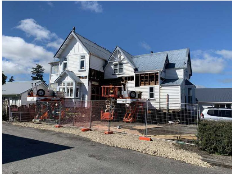
Illustration 6: Vicarage uplift from Church Street (4rd April 2022 Abbeyfield).
