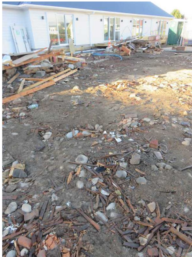
Illustration 15: Artifact scatter 2 facing towards new residential units prior to excavation (8th April 2022).
