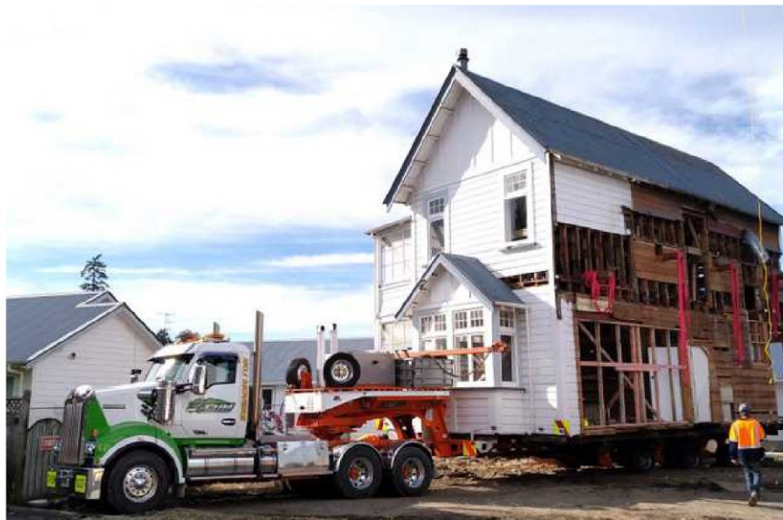
Illustration 7: Building removal in progress (4th April 2022 Chessa Stevens).
