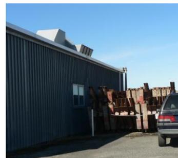
*Example of roof services requiring specific design (colour and location). Note unacceptable storage alongside building)*
